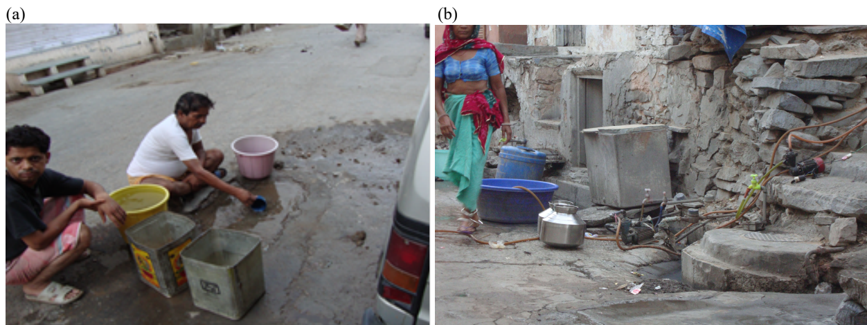
Fig. 2 (a) Low Water Supply Pressure and (b) Leakage due to accident vandalism
